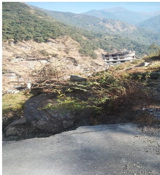
Sinking Naga Nagmore
